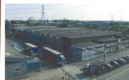
AGM Battery Manufacturing Plant, Newport, Wales, UK
