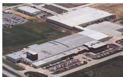
AGM Battery Manufacturing Plant, Warrensburg, MO, USA
